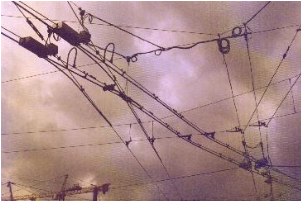
A modern switchgear for trolley buses in an Arnhem bus station, picture ScanTech Development
