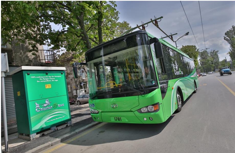
Charging station, 660V DC to 585V DC
