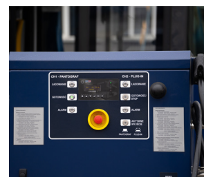
ABOVE: Pantograph charger console. SOURCE: Open Charge Alliance
